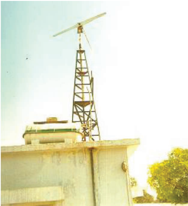
Fig. 1 Two bladed 500 watt horizontal axis wind turbine
