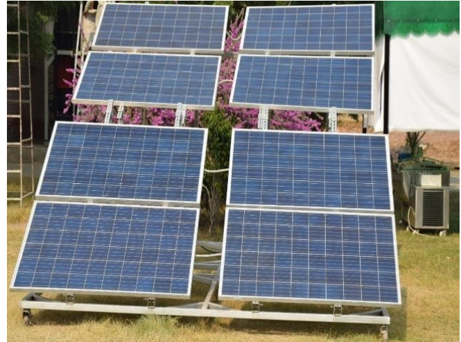
Figure 4. Solar PV panels of 2kW.
