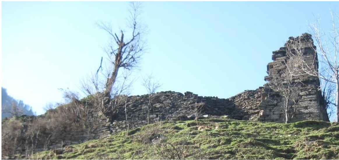
Figure 1. Southern side of the temple lapsed due to the weakening of foundations by floods
