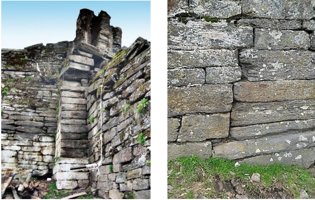
Figure 4. Earthquake jostling in Šarda Complex a. joint of stair case with the main court b. outside view of the base of the northern wall
