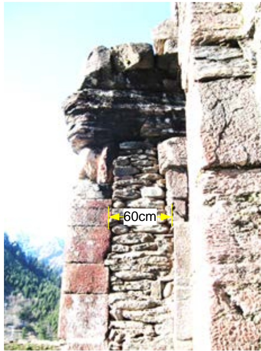
Figure 14. The remaining pillar of the canopy to the door from southern side in front of door. These repairs have cement used in some instances.
