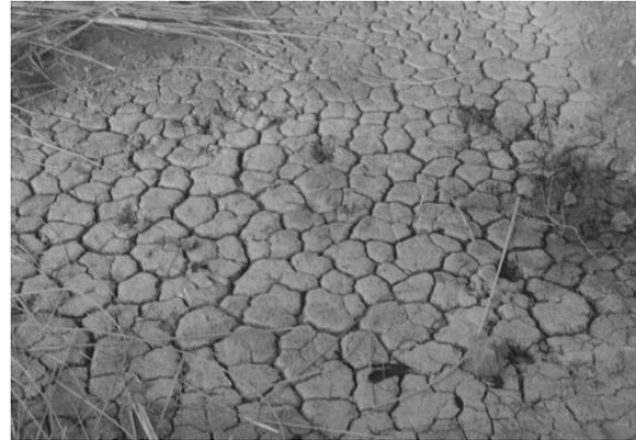
**Fig.2** Typical appearance of expansive soil with ground cracks [7].
