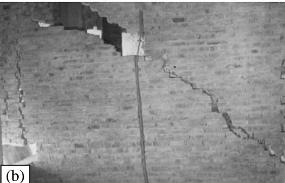
**Fig.1** Damages in structures founded on swelling soils: (a) Cracks in residential building that have been repaired; (b) Failure of partition wall due to diagonal expansive crack [7].
