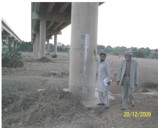
**Figure 7:** Stream Gauging Station at Super Highway Bridge across river Malir
