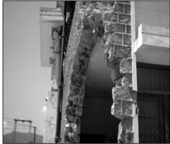
**Figure 3:** Corner joint failure of bonded masonry in Bagh
