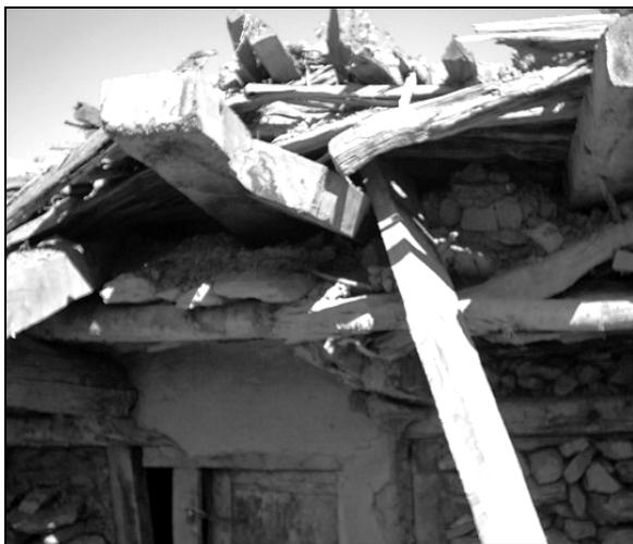
**Figure 2:** Thick layer of mud collapsed in earthquake
