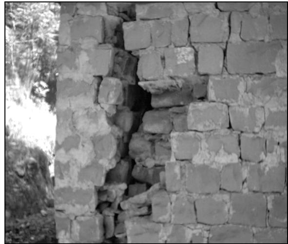
**Figure 4:** Typical corner joint failure of a house in Bagh
