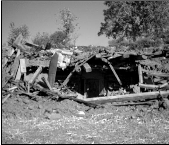
**Figure 1:** Collapsed house in Balakot with heavy roofing.
